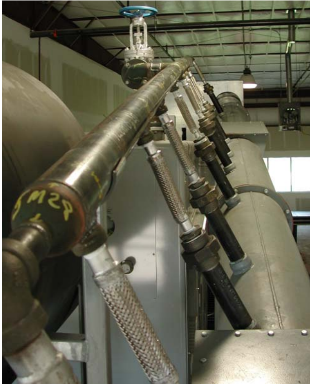
Figure 1. Mobile pilot plant inoculation and pile-building trailer: Decontamination steaming conveyor alongside of boiler.
