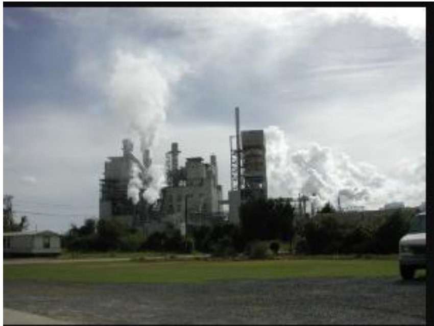
International Paper Company, a pulp mill that makes fluff pulp for use in absorbent products with the kraft process (USA).
