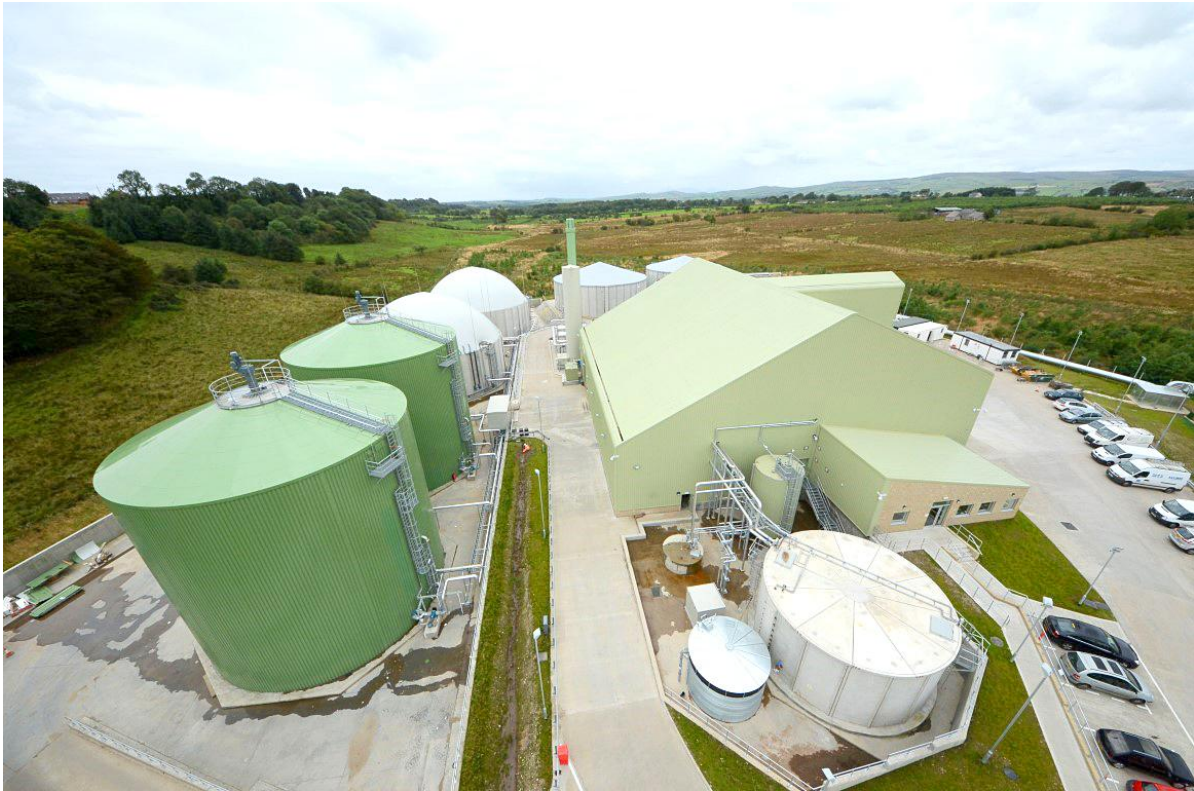
View of a working plant in Scotland
