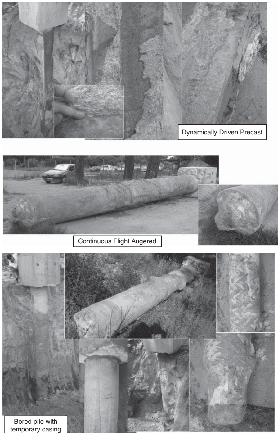
Figure 8.41 Some of the differences in the three types of piles after extraction
