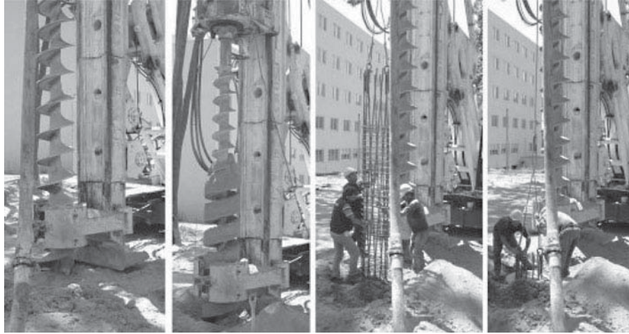
Figure 8.39 Installation of CFA pile
