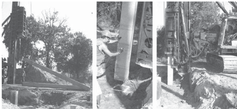
Figure 8.40 Installation of precast concrete driven pile
