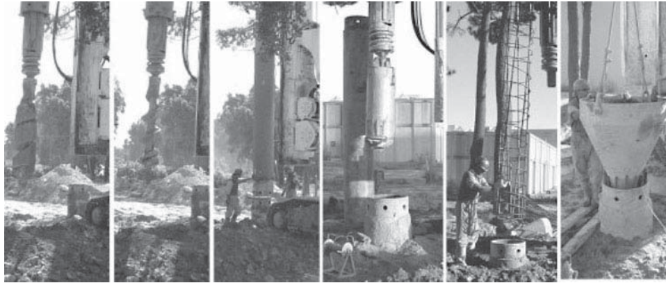
Figure 8.38 Installation of the bored piles with temporary casing
