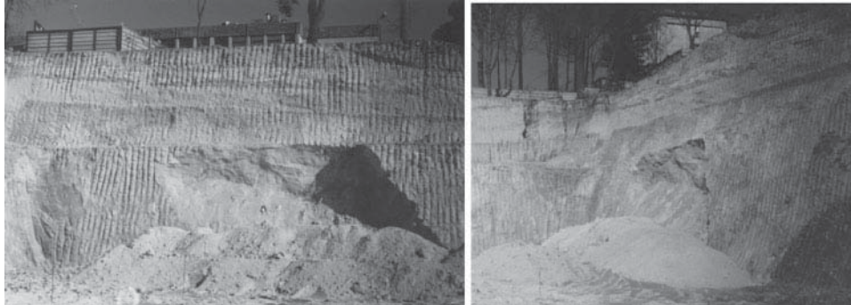
Figure 8.2 Parent rock with potentially unstable weak features (Porto, Portugal)
