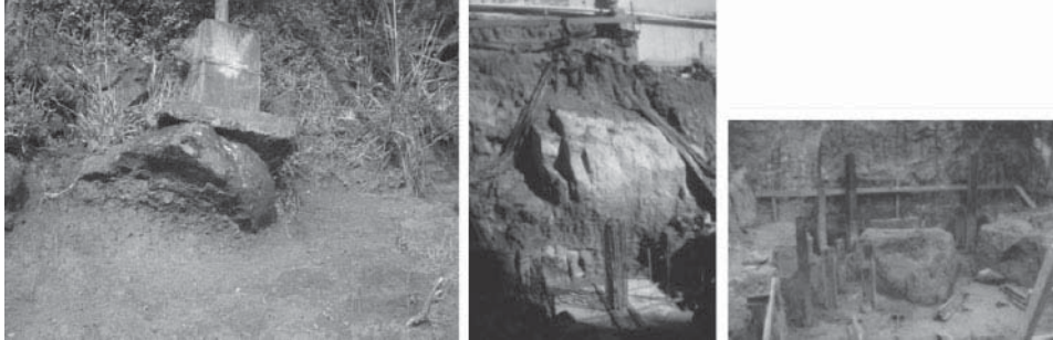
Figure 8.1 Uncertainties due to heterogeneities of residual profiles (After Milititsky et al. , 2005)
